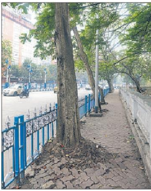
The roots of a tree covered with paver blocks on the footpath near American Center
